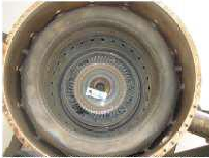
Photo No. 25, Compressor turbine in-situ and combustion liner
